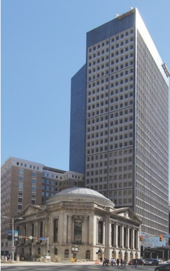
Photo: Courtesy of Geis Companies and Foss and Company Inc.
